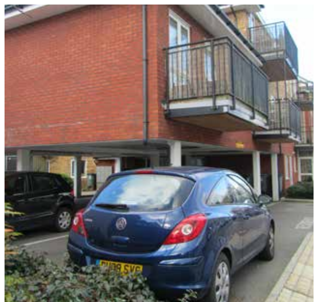
Covered car parking spaces located at ground floor level
