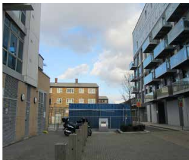
Servicing area provides a less active frontage overlooking a car park and the rear of neighbouring buildings.
