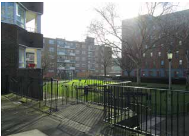
For smaller schemes, the absence of any shared amenity space may not be an issue if there is good provision nearby.
