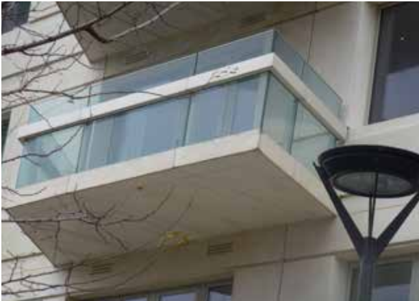
The fabric of the building remains in good order following completion.
