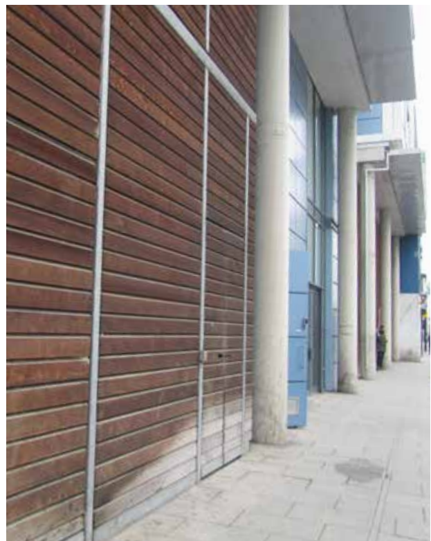
Refuse storage areas can result in a blank street frontage if positioned at the front of the building.
