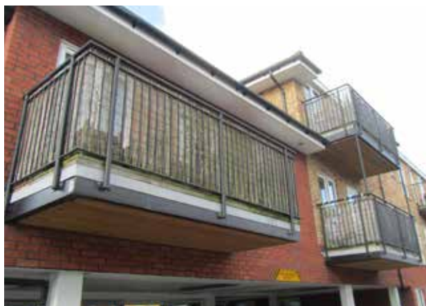
Additional screening provided by an occupier around a balcony.
